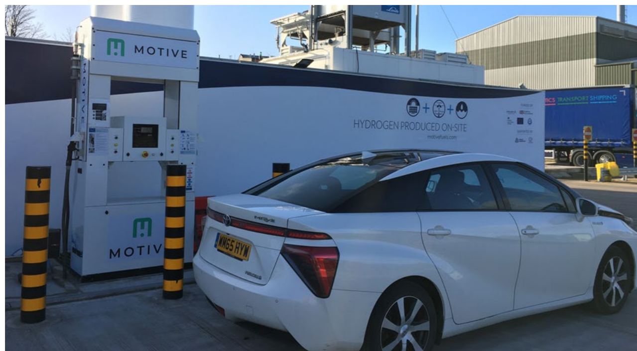
Hydrogen refuelling station at Tyseley Energy Park in Birmingham.
